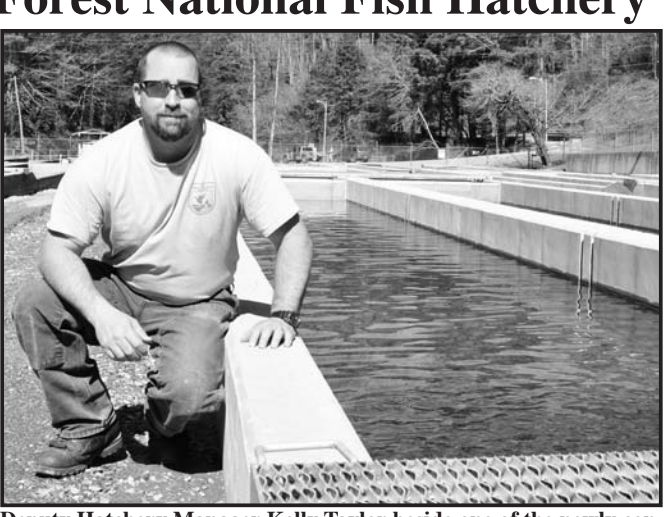
Deputy Hatchery Manager Kelly Taylor beside one of the newly constructed raceways.
