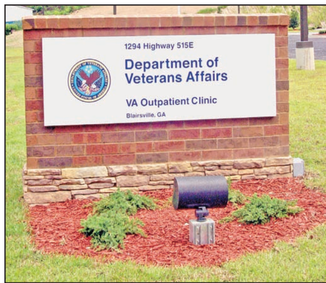
The VA Outpatient Clinic in Blairsville is nearing completion. Officials say the next step is a construction inspection. The clinic, which also serves Towns, is slated for a September opening. Photo/Norman Cooper
